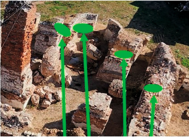
Fig. 9. Intersections of local maxima under the ruins of the Transfiguration Cathedral at a depth of 1.5–2.0 m indicating possible cavities under the altar and in the area of the columns.
