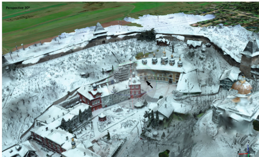
Fig. 4. General view of the Holy Dormition Pskovo-Pechersky Monastery obtained by aerial photography. The arrow shows the entrance to the cave temple.
